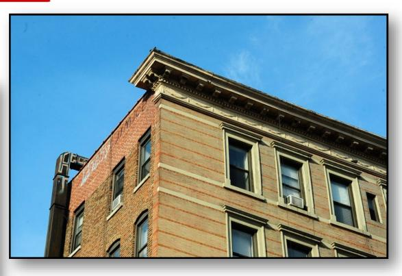
DECORATIVE CORNICES: Not considered "usable" as part of the Perimeter Access Landing Areas. Calculations must begin on the main rooftop level and after the termination of the façade wall.
