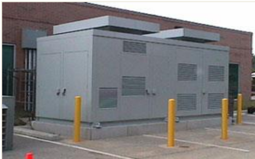
New York City Transit Off-peak electric storage for a bus refueling station, using a sodium-sulfur battery system
