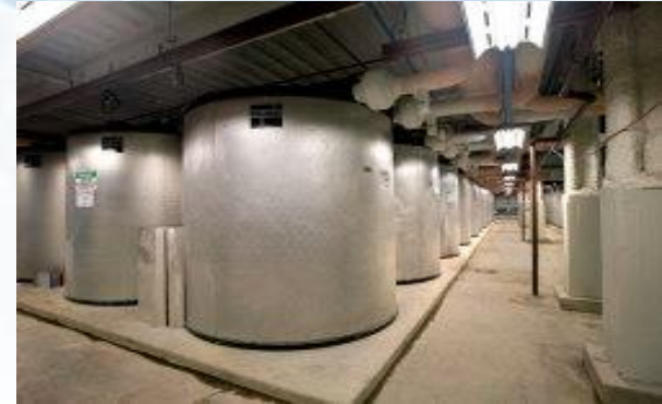
Calmac Manufacturing, NYC Ice storage system for permanent peak reduction
