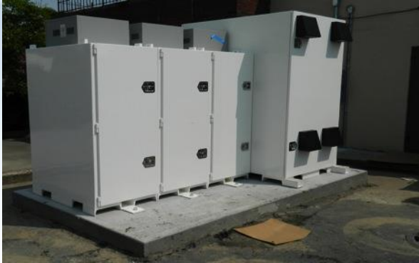
Green Charge Networks, NYC 100 kW lithium-ion system for demand charge management
