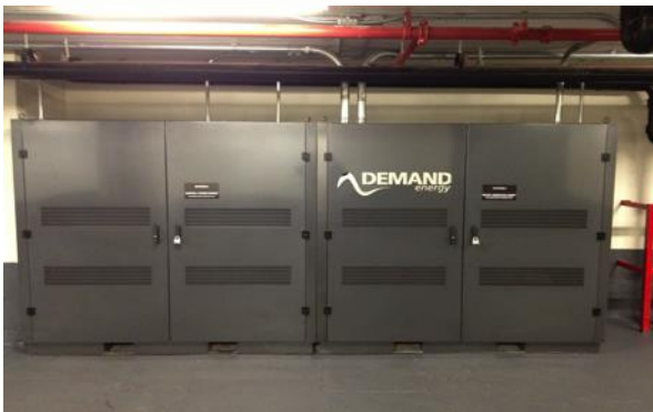
Demand Energy, NYC 225kW lead acid storage system for energy management & backup
